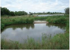
large particles are deposited as the water spills over a weir into the constructed wetland. Plants filter pollutants and nutrients in the wetland and then, the filtered water is controlled and released slowly through an inline water level control structure. A stacked stone weir was installed at the downstream end of the wetlands for flow rate control.
