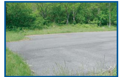
New pervious asphalt parking lot provides needed citizen access while demonstrating an innovative BMP.
